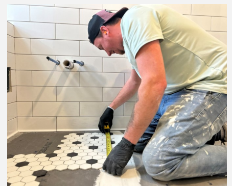
Zach Ramberg installs tile in the wheelchair accessible restroom on March 25.
